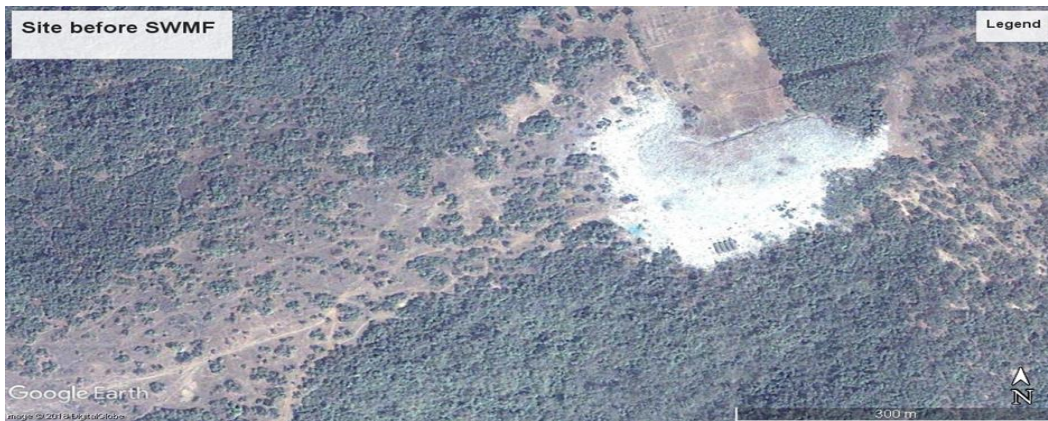
Figure 11. Google Earth Image before the SWMF at Saligao
