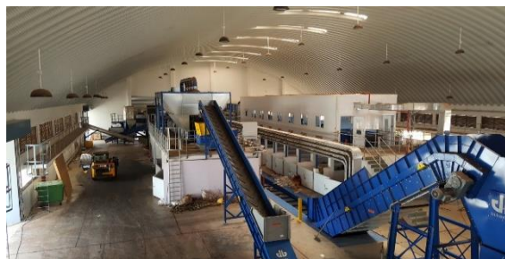
Figure 5. Inside Material Segregation and Recovery Facility
