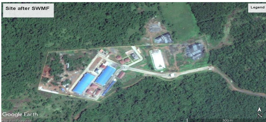
Figure 12. Google Earth Image after the SWMF at Saligao
