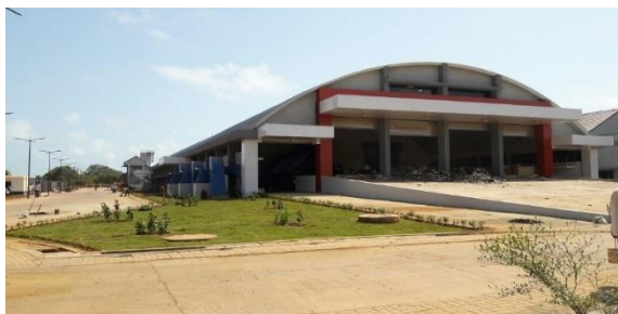
Figure 4. Tipping Floor Shed
